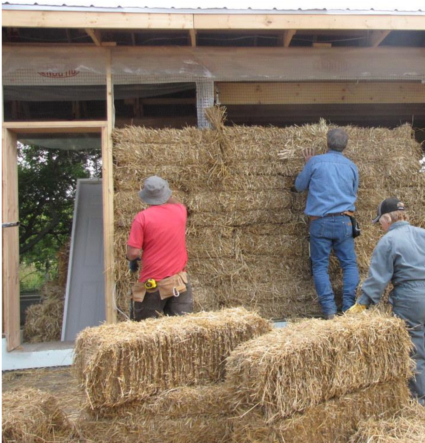
Volunteers help construct a straw bale home in Craik, SK.
