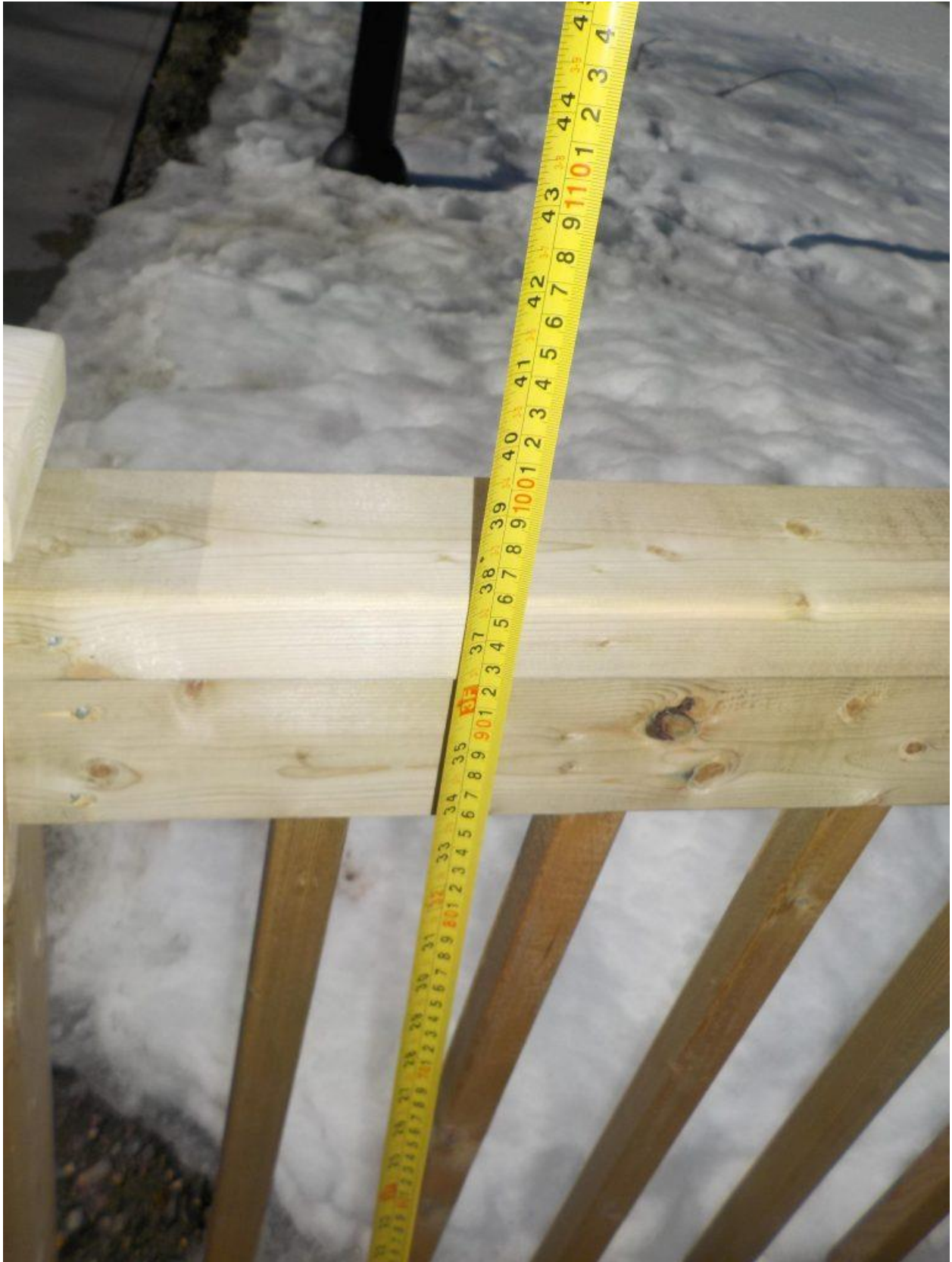
One of our inspectors verifies the height of an exterior guard. It's 96 cm high: is that
