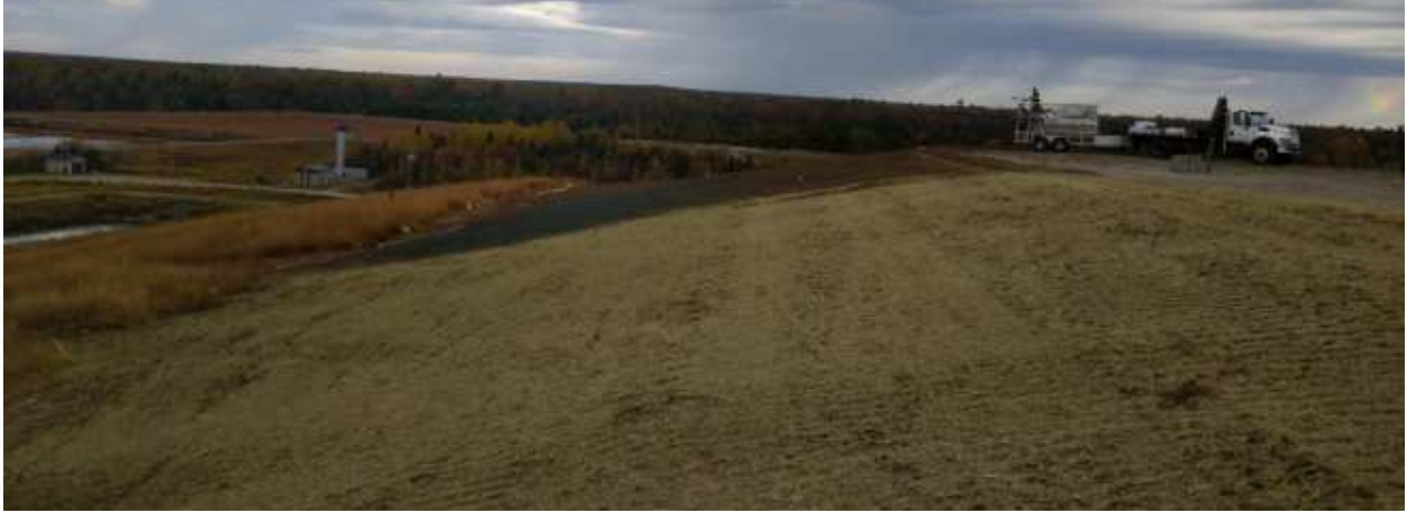
Final capping being completed on the cell complex south slope.
