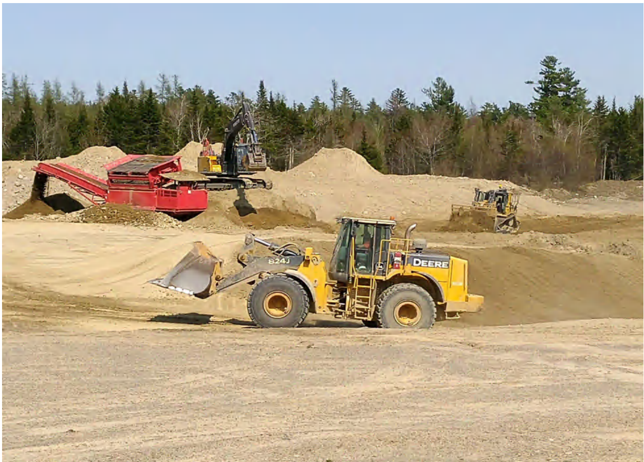
Screened clay is required for the landfill capping as well as the cell liner construction.
