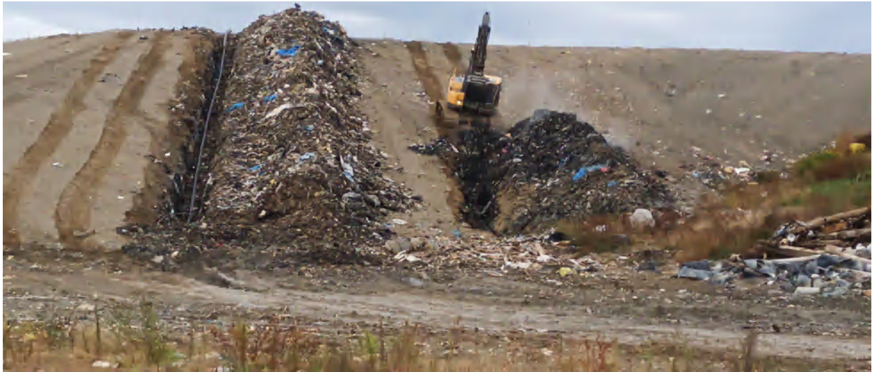
Two additional LFG wells were installed and will be connected to the collection system.
