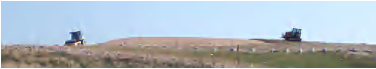
Final capping being completed on the cell complex south slope.
