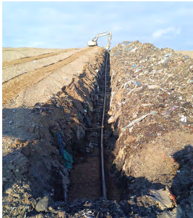
An LFG well using perforated piping being installed to collect subsurface landfill gas.
